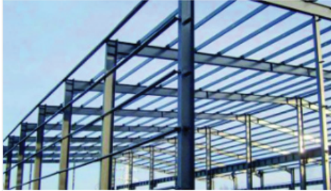
Designing & Manufacturing Steel Structures
